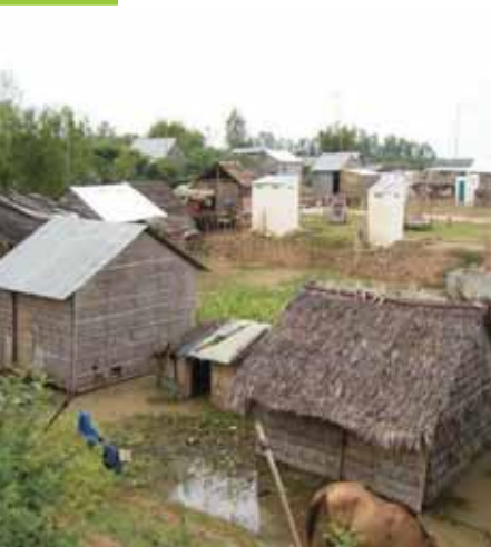
Resettlement site of Highway 1 flooded in rainy season.
