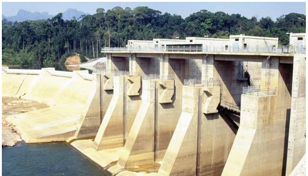
Theun-Hinboun Hydropower Dam. Photo: International Rivers
