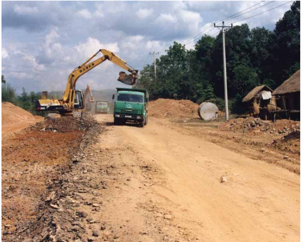
Route 9 construction. Photo: Jonathan Cornford/OxfamAUS
