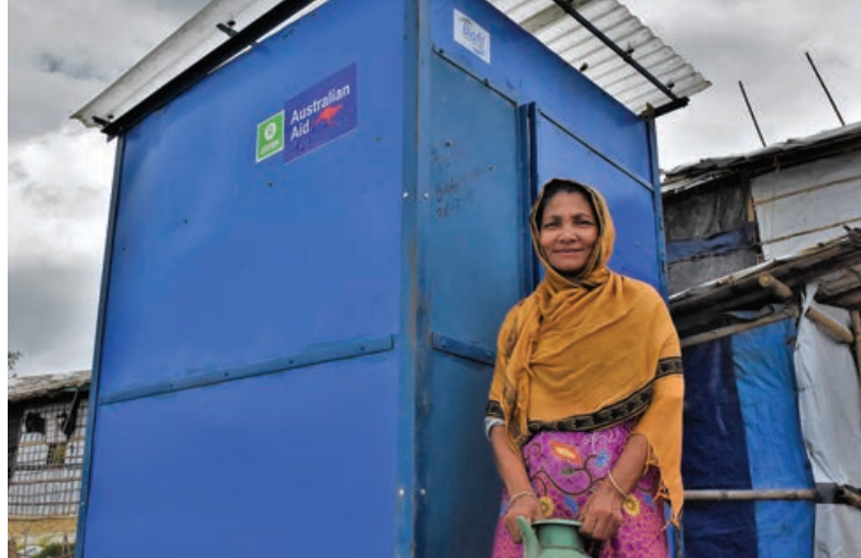
Cox’s Bazar, Bangladesh: Camp resident stands next to Biofil latrine, which uses worms to decompose fecal waste. Photo: Maruf Hasan/OxfamAUS.
